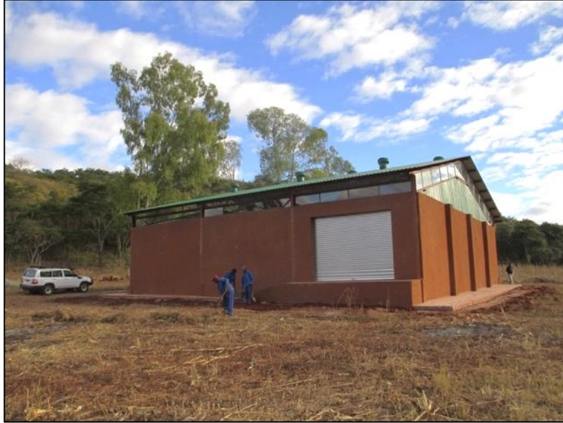
Figure 5: Example of typical shed suitable for production (Credit: G. Le Breton)
